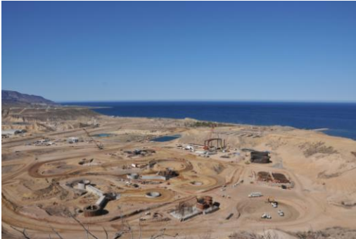
PROCESS PLANT CONSTRUCTION AT BOLEO – SEP 2011
