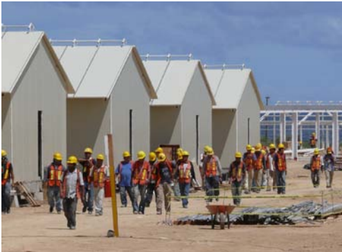
CAMP CONSTRUCTION - PHASE 1
