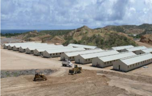
CAMP CONSTRUCTION - PHASE 1
