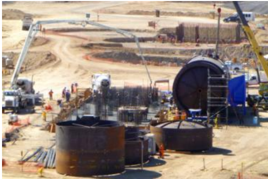
ACID PLANT CONSTRUCTION– NOV 2011
