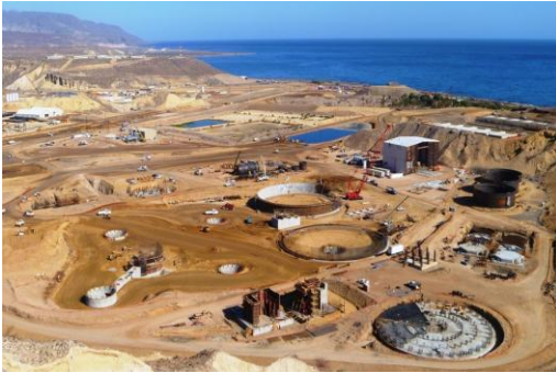
PROCESS PLANT CONSTRUCTION AT BOLEO – NOV 2011
