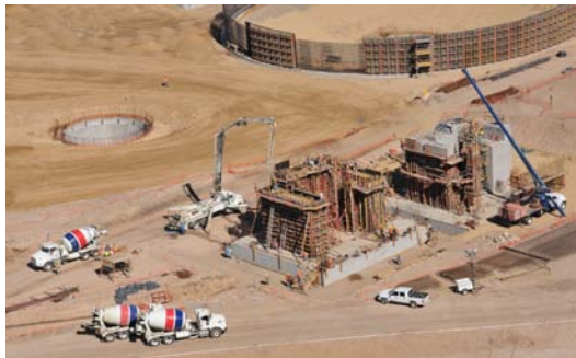
SCRUBBER AND BALL MILL FOUNDATION– NOV 2011
