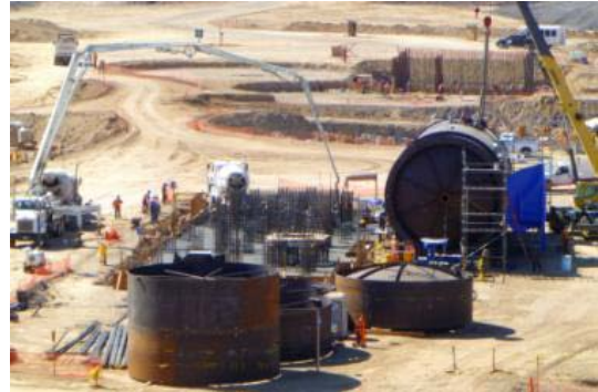
CONSTRUCTION OF THE ACID PLANT– NOV 2011
