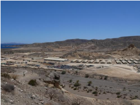
CAMP & PLANT OVERVIEW – APRIL 2011
