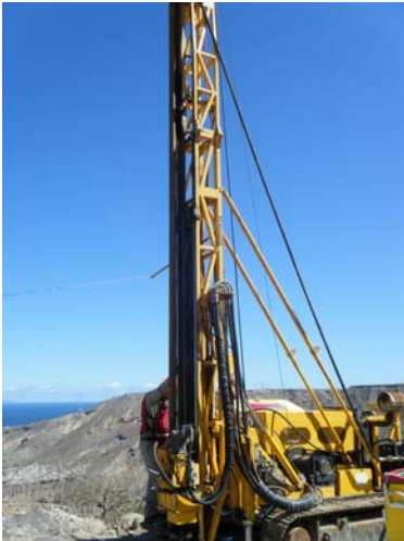
DRILLING PROGRAM – FEB 2012
