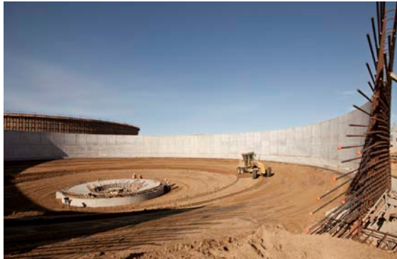
CONSTRUCTION OF CCD THICKENER WALL— JAN 2011
