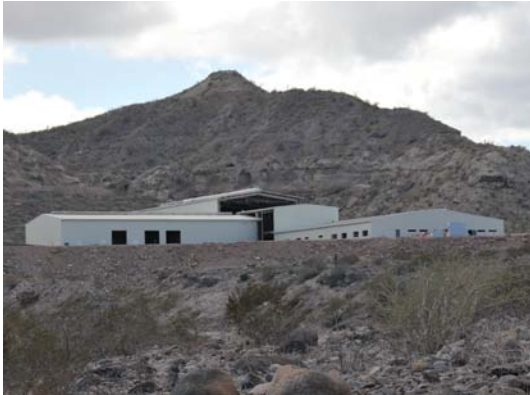
MINE MAINTENANCE FACILITY (MMF) BUILDING - JAN 2011
